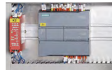
Siemens PLC Control
